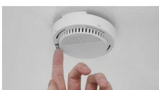
Since the smoke detector is the best way to save lives, it is important to regularly check that it is working properly by pressing the test button until the audible sound signal is heard. That should occur within seconds.
