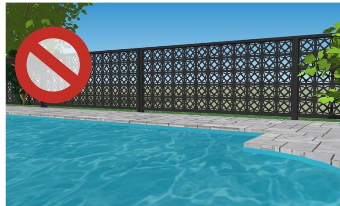
Example of an ornamental fence that can be easily climbed.
